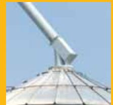
**2.** Filling box on the inner roof prevents grain crushing, eliminates the abrasion on the inner roof and it is capable of self-cleaning.
